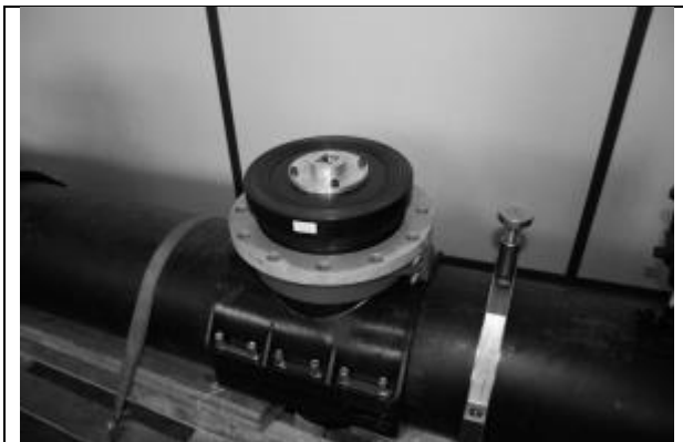
Fig. 54 - Removal of POLYSTOPP® 10" Valve, reinforcement collar and valve support
