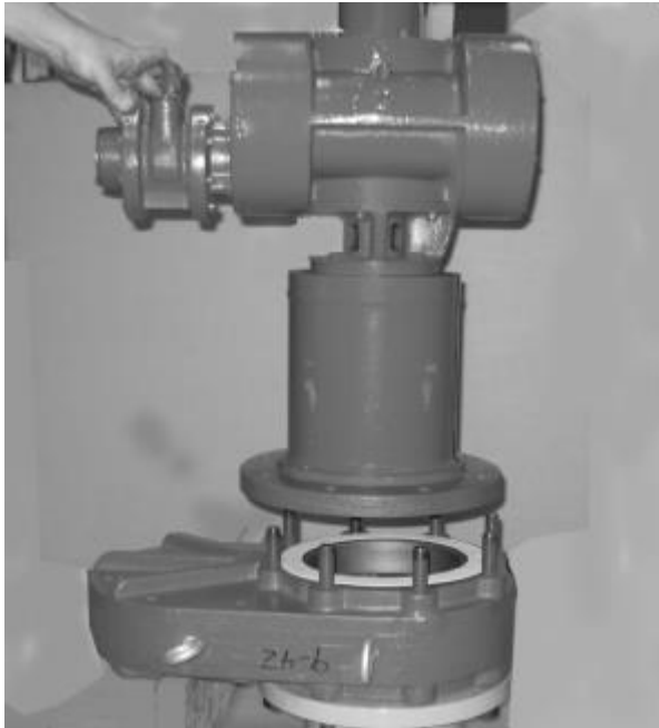
Figure 22. Install T-203 Tapping Machine (valve design will be changed after September 2019)
